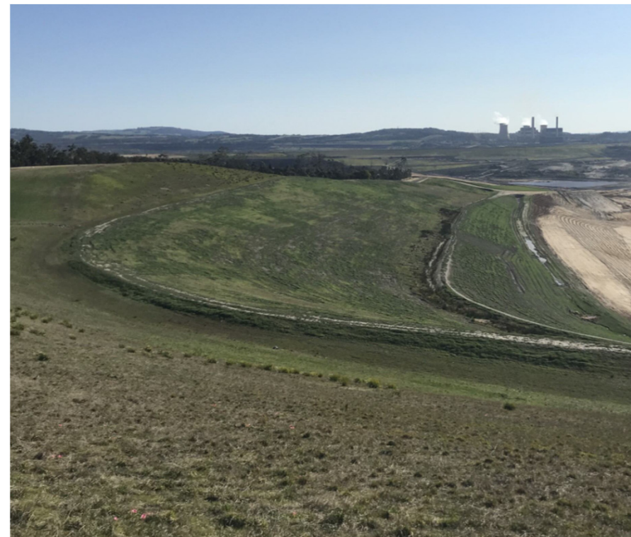
Figure: Progressive rehabilitation completed at East Field Extension Southern Batter
